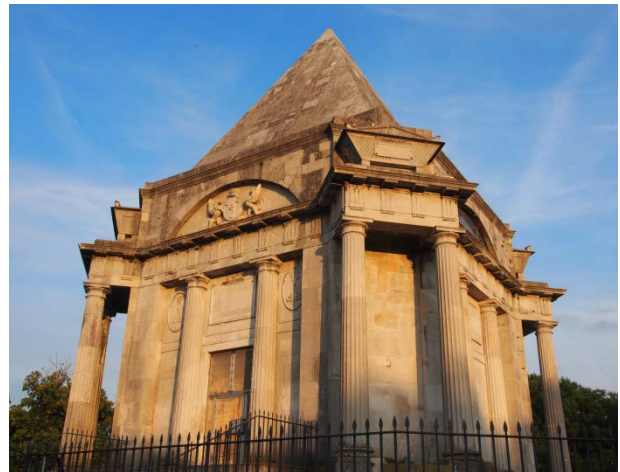
The Darnley Mausoleum in Cobham Park has been rescued from dereliction and restored. It is now occasionally open to the public.
