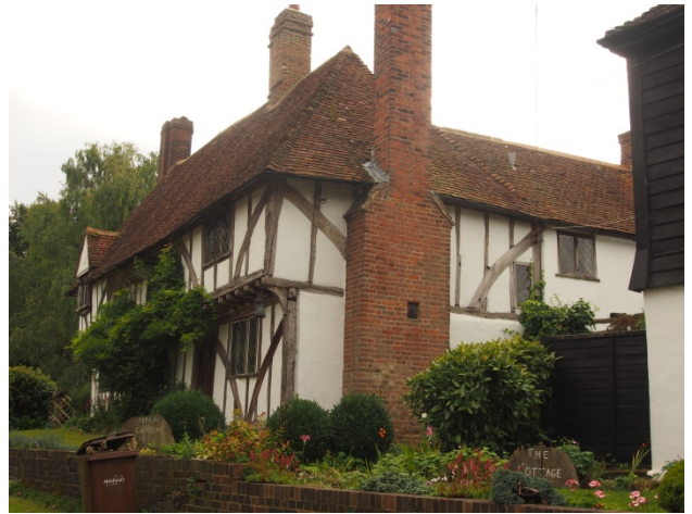
Timber-framed buildings in Upper Bush Conservation Area
